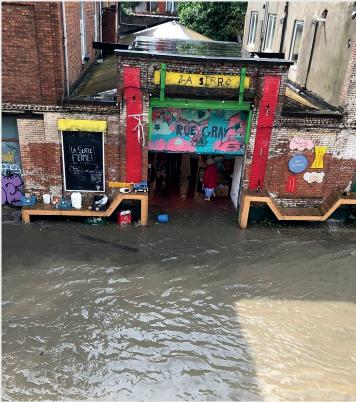
Figure 2: Flooding in the street in front of the community space (BX1, July 9 2024)
